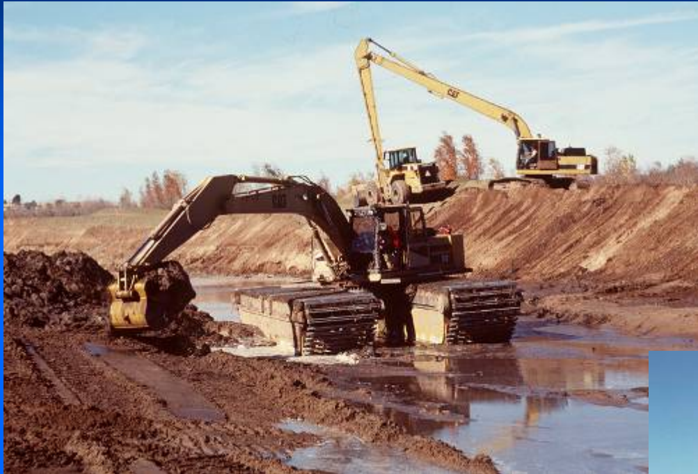
Excavation of new backwaters
