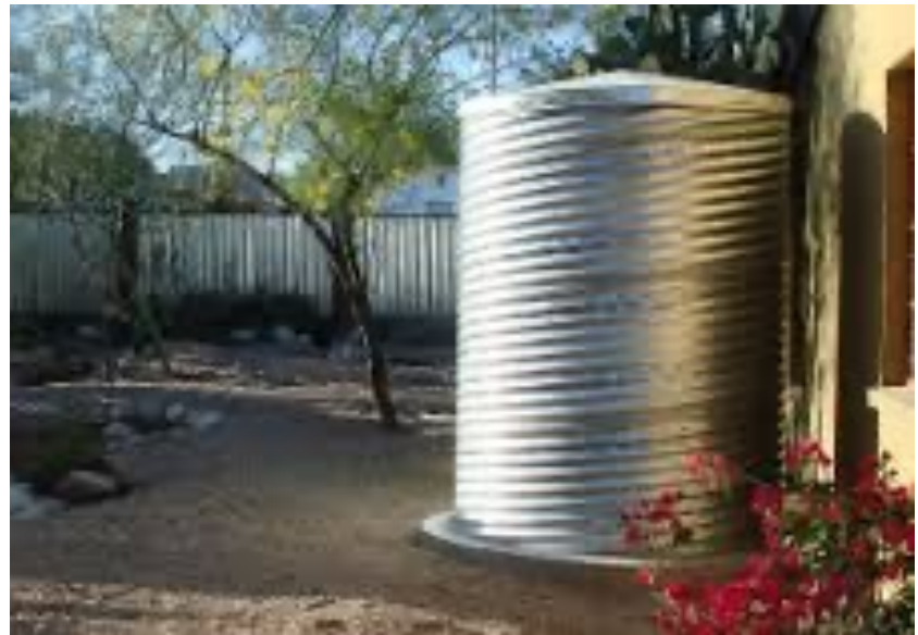
Active rainwater harvesting system
