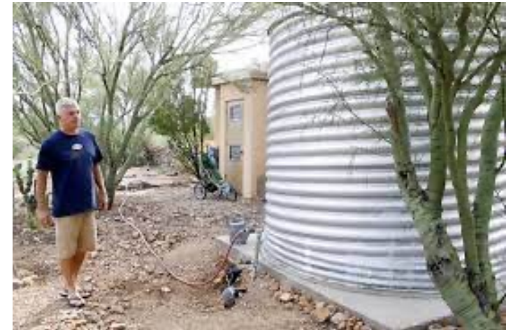
Active rainwater harvesting system
