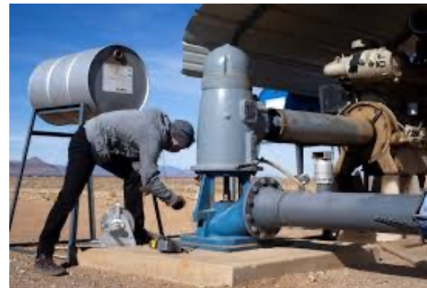
Electric water well
