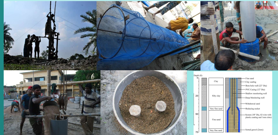
Construction of Recharge Wells in Coastal Bangladesh
