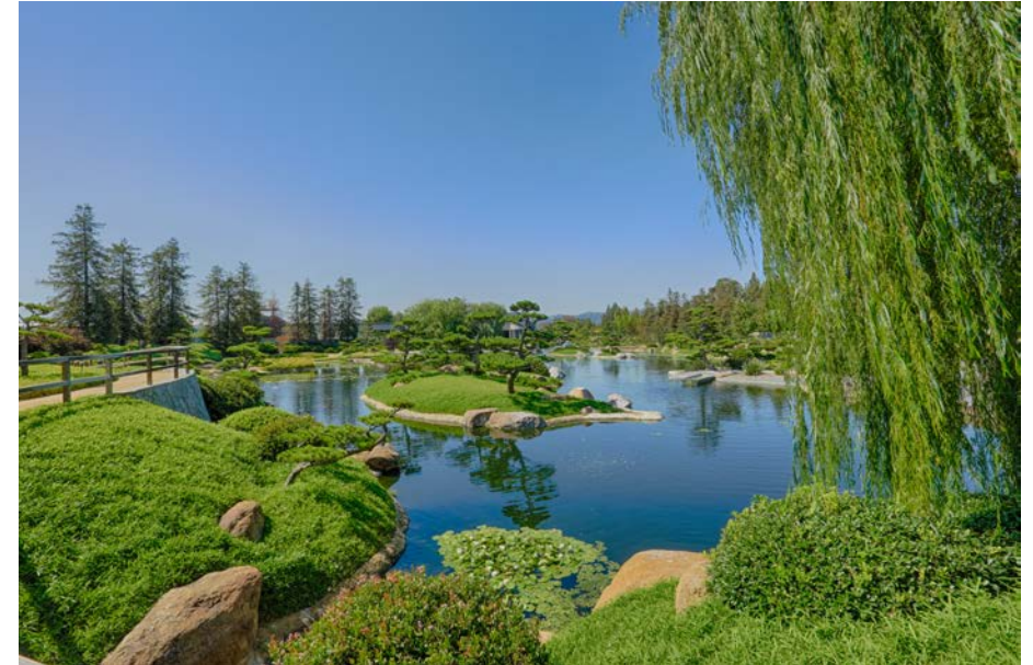
City of Los Angeles, Sanitation & Environment operates the Donald C. Tillman Water Reclamation Plant, which provides recycled water to customers in the San Fernando Valley and irrigates its onsite Japanese Garden
