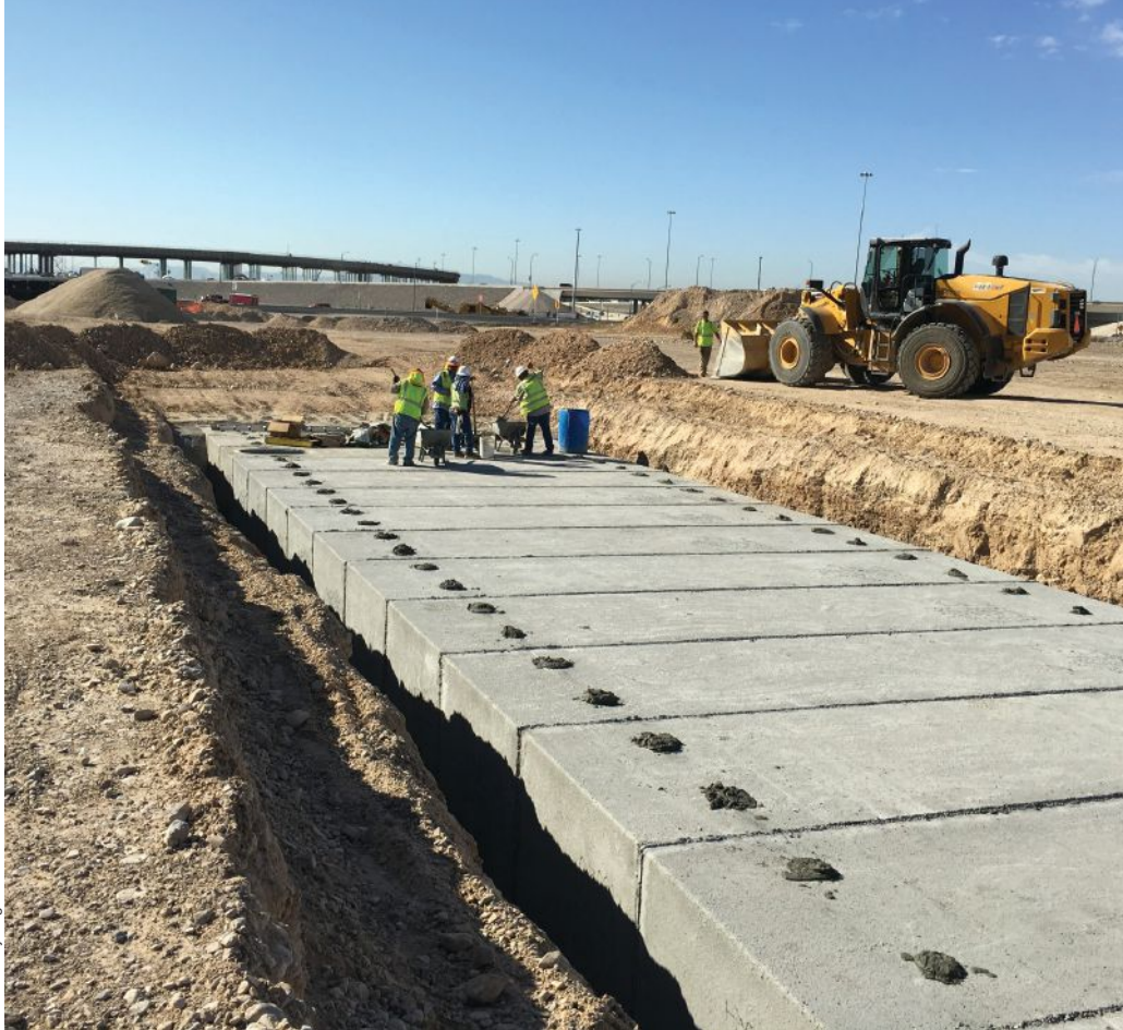
Culvert installation under the Centennial Bowl
