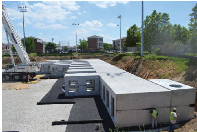
StormCapture system installation
