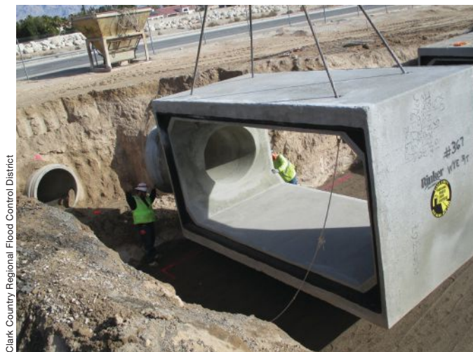
Culvert installation under the Centennial Bowl
