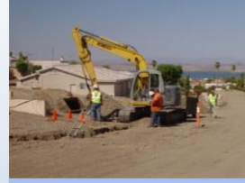
Converting city from septic to sewer Lake Havasu City
