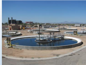
Water Reclamation Facility City of Casa Grande
