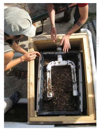
Woodchip bio-filter to trap grease and food particles from a kitchen sink. The top half of the inlet pipes has been cut off to allow the greywater to flow over the edges and distribute into the wood chips.
