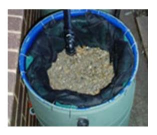
An example of a sand filter system, Basically it is made up of a thin layer of gravel topped off with a much thicker layer of sand within acontainer (old plastic barrel or drum). Coarsly filtered water passes through the sand being finely filtered.
