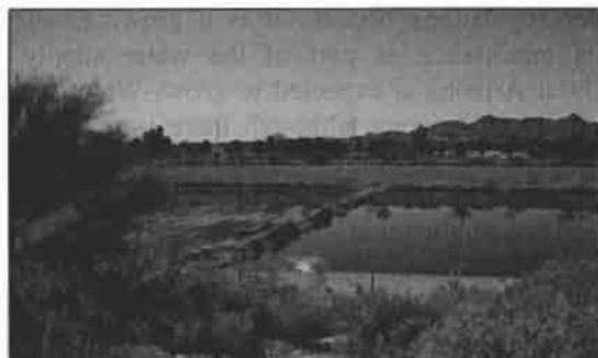
Figure 4. Effluent recharge basins at the Sweetwater Wetlands reclamation facility (Courtesy of Deirdre Brosnihan.)
