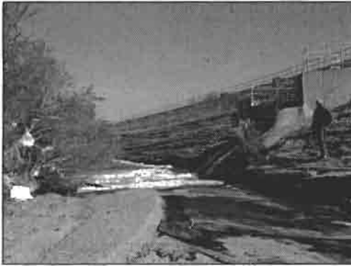
Figure 2. Outfall of regional wastewater treatment facility (Courtesy of Pima County Regional Flood Control District.)
