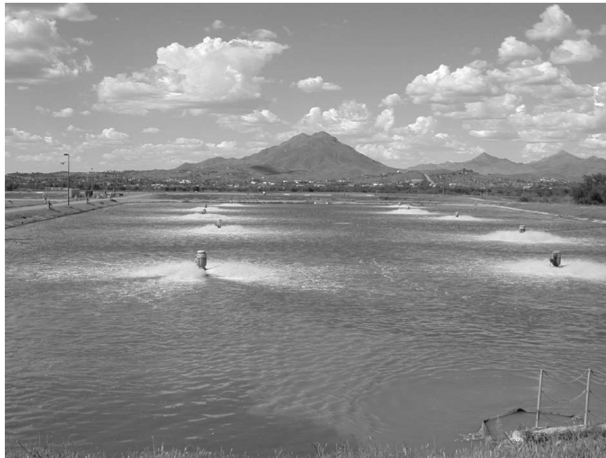
Aeration ponds at treatment plant
