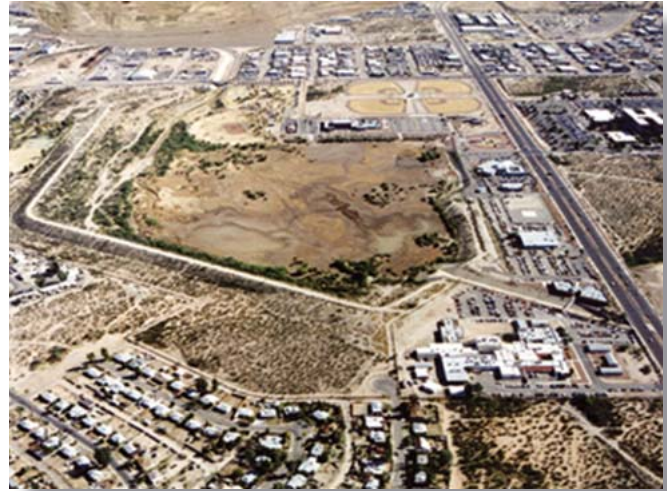
Ajo Detention Basin
