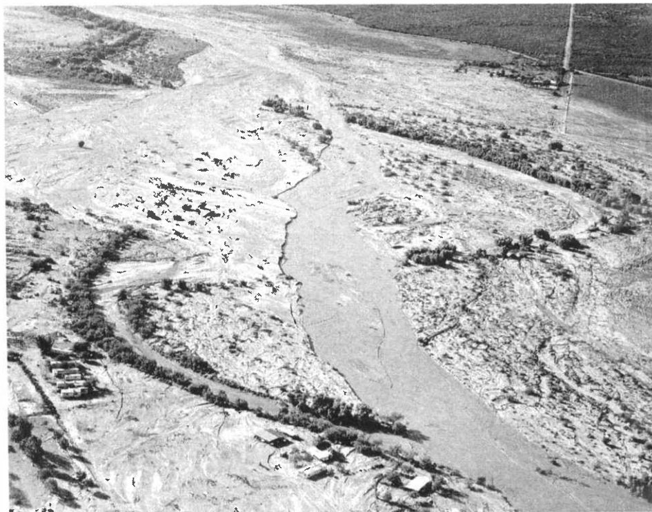
"Should we concrete the banks of the Santa Cruz River?" is the topic of a slide show to be presented by Ed McCullough at an October 12 Sierra Club meeting, to be held 7:45 p.m. in Room 201, PAS Building, University of Arizona, Tucson. Above is the rampaging Santa Cruz River cutting off a meander channel (note trees along the original channel) during 1983 flooding. (Photo: P. Kresan)
