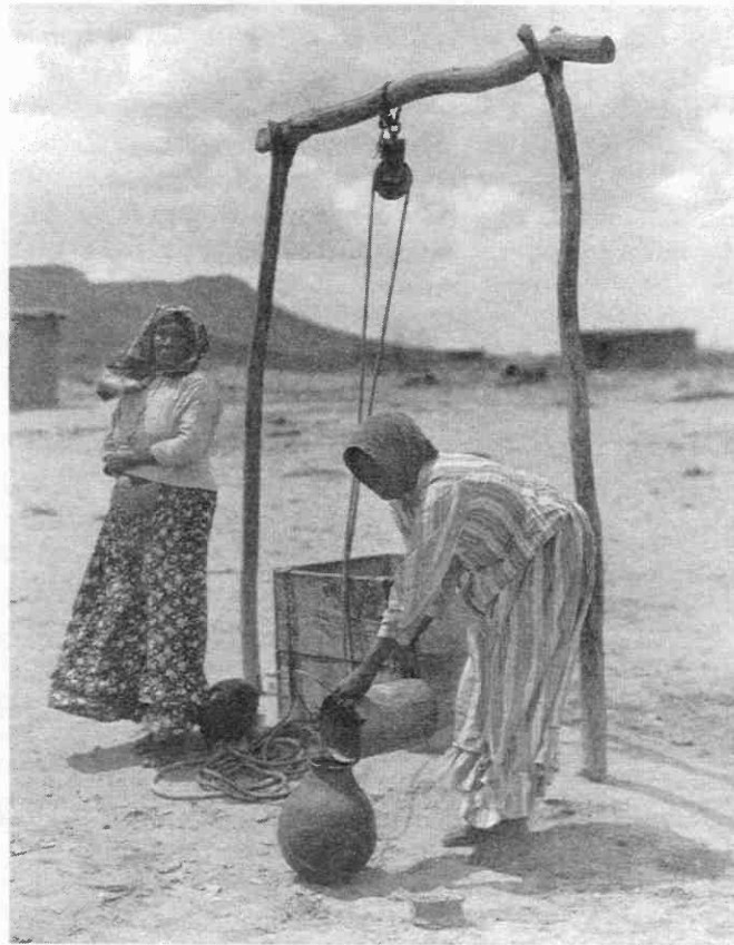
Papago (Tohono O'odham) women fill their ollas from a hand-dug well on the San Xavier District of the Tohono O'odham Reservation southwest of Tucson. The date is uncertain, but the length of rope indicates very shallow groundwater. Today, depths to groundwater beneath the District average several hundred feet.
