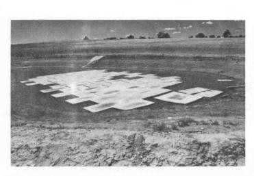
Figure 2. Compartmented pond reservoirs at Black Mesa are outfitted with floating polyurethane rafts to cut evaporation.
