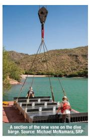
September 2013, engineers at the Salt River (SRP) Project successfully executed a unique underwater method to repair a damaged intake structure for Horse Mesa dam's hydroelectric Unit 4. In June 2012, the collapse of a guide vane inside the penstock intake-that is, the huge pipe that passes through Horse Mesa dam from Apache Lake into the generating unit below on the Canyon Lake side-shutdown Unit 4 and the 119 megawatts of electricity generated by its pump-back unit. To repair the damage SRP
