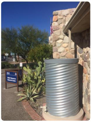
Water harvesting containers capturing rain water from roof downspouts
