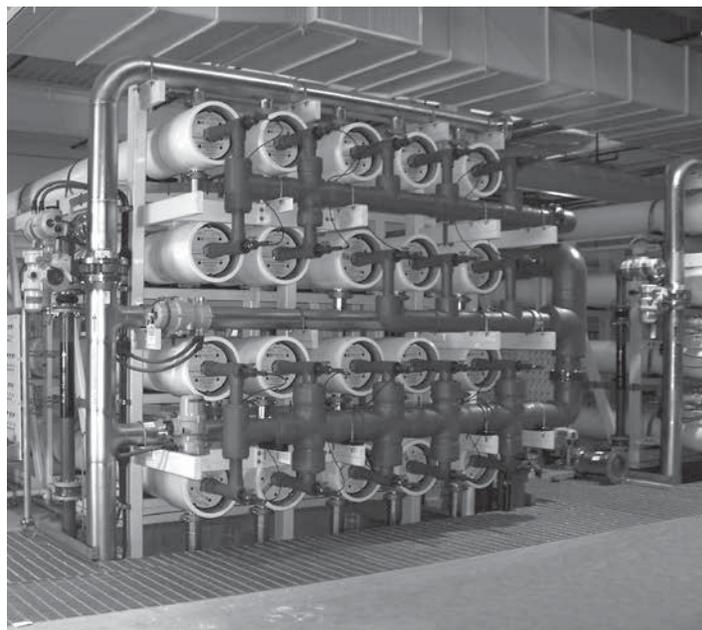
**Figure 3:** Reverse osmosis train removes persistent chemicals from effluent at the Scottsdale Water Campus
