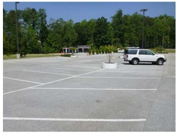
Figure 3.4. Pervious concrete pavement. For more information regarding pervious concrete: <u>http://acpa.org/PerviousPave/</u>
