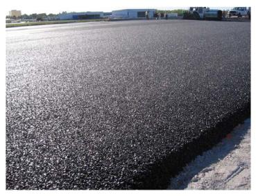
Figure 9.12. Completed porous asphalt installation.
