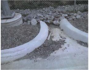
Figure 9.6. Example of a curb cut-out.
