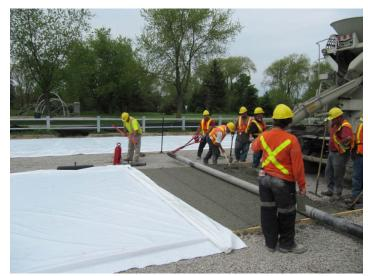
Figure 9.13. Pervious concrete placement, jointing and curing.
