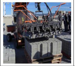
Mechanical installation of interlocking concrete block pavers.
