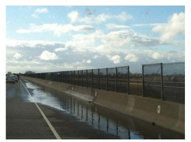
Figure 1.1. Ponding on highway shoulder.
