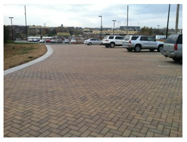
Figure 9.14. Typical permeable interlocking concrete pavement installation.
