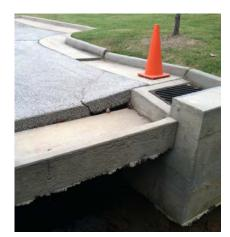
Figure 9.15. Pavement failure due to water erosion.
