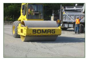
Figure 9.7. Appropriate compaction equipment for open graded aggregate.
