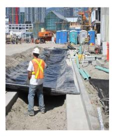
Figure 9.1. Installation of a geomembrane.
