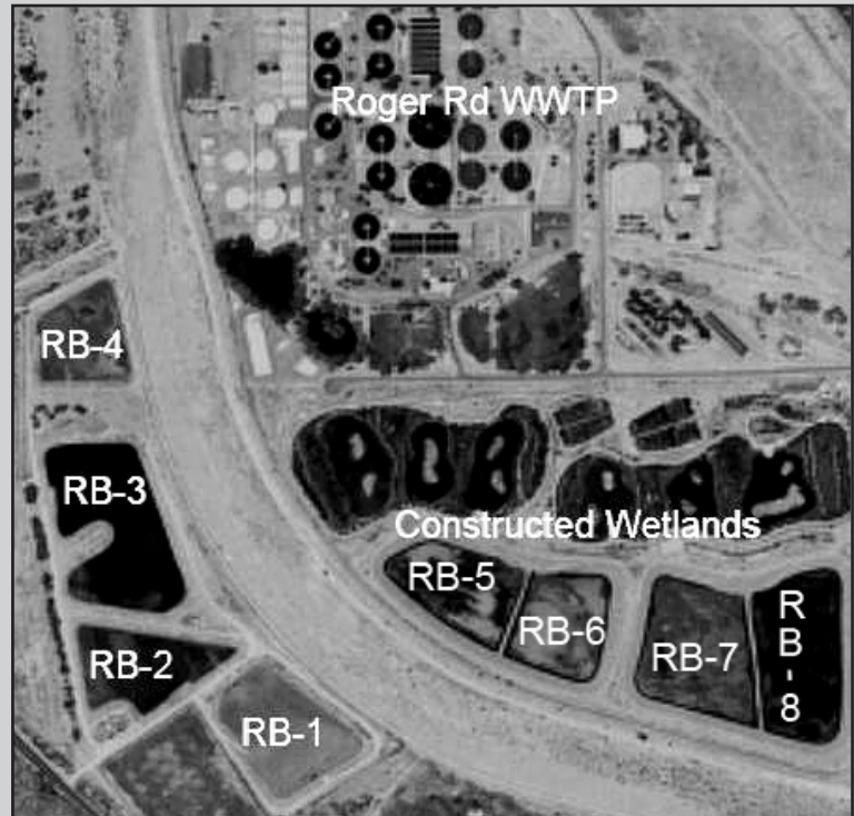
Sweetwater Recharge Facility in Tucson, with eight recharge basins (RB-1 to RB-8) and constructed wetlands
