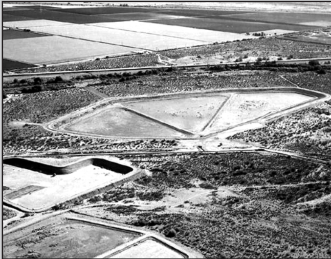
Above are the triangular-shaped basins of the Lower Santa Cruz Recharge Project. In the foreground are Avra Valley Recharge Project basins.
