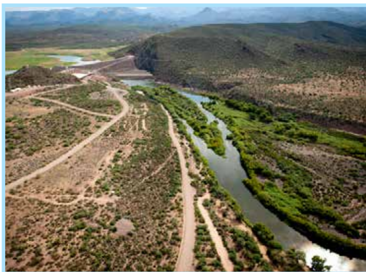
Horseshoe Dam, an earth-fill structure 194 feet high on the Salt River in Arizona. Source: U.S. Bureau of Reclamation, Andrew Pernick.
