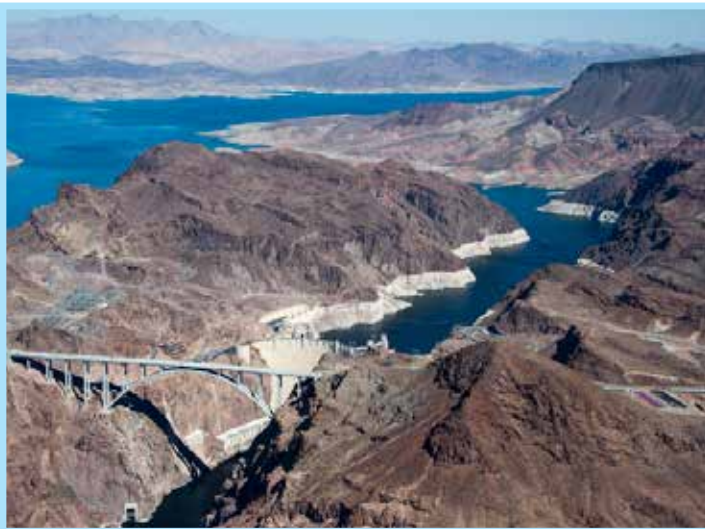
Lake Mead. Source: Central Arizona Project.
