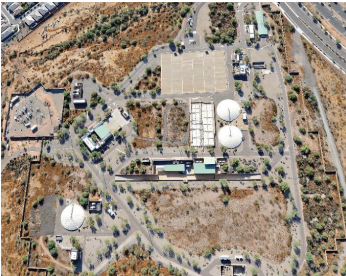
Cave Creek wastewater treatment plant site for planned Advanced Water Purification plant. Source: Phoenix Water Services
