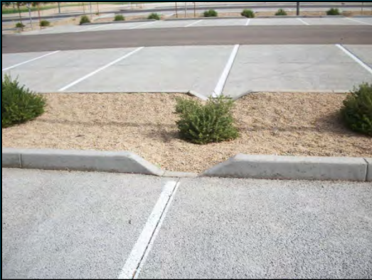
Pervious concrete at Phoenix Manzanita Park Parking Lot
