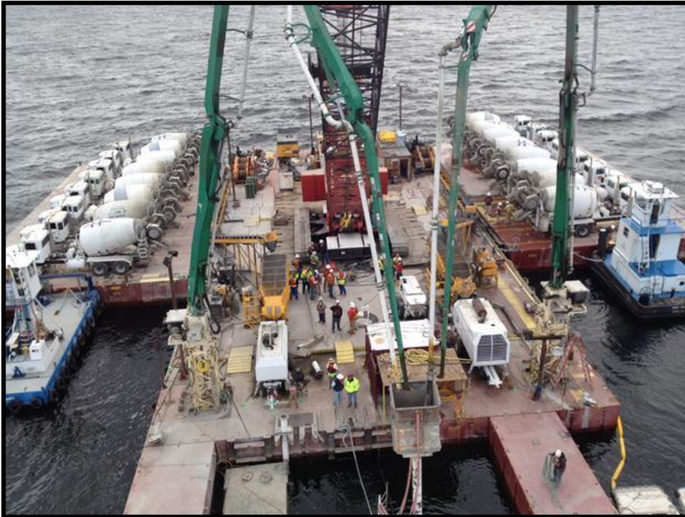
Cement trucks for intake structure placement
