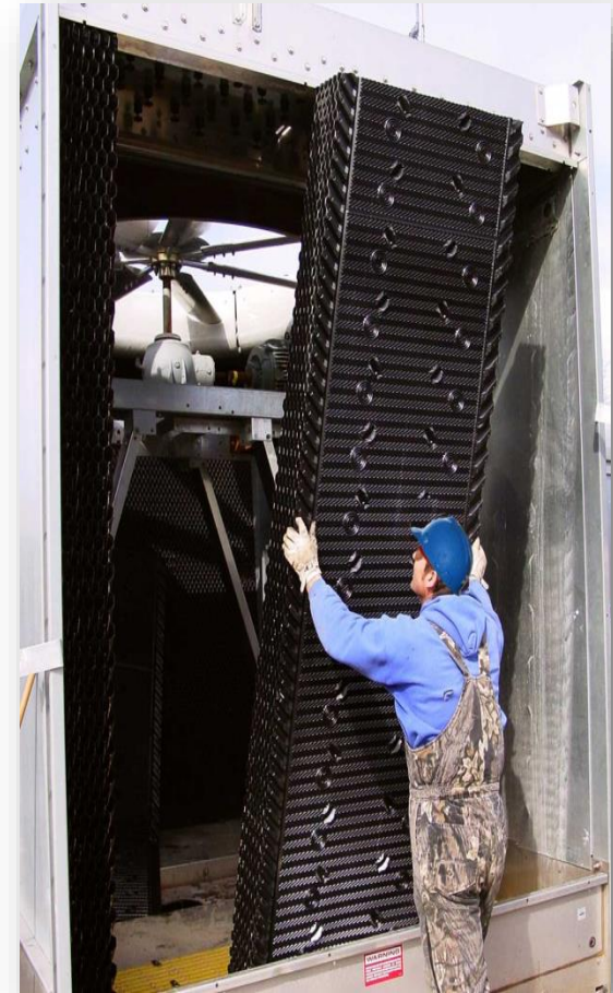
Worker updating a cooling tower
