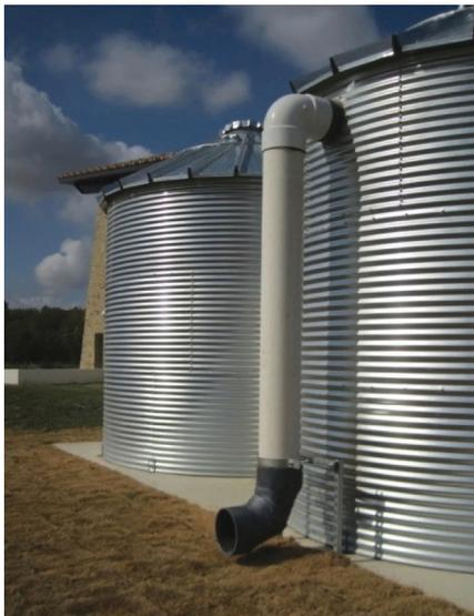
**Figure 9.12** Tank overflow pipe
