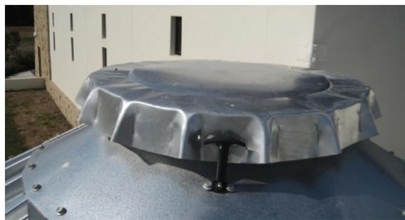
Figure 9.10 Round tank access port with locking lid
