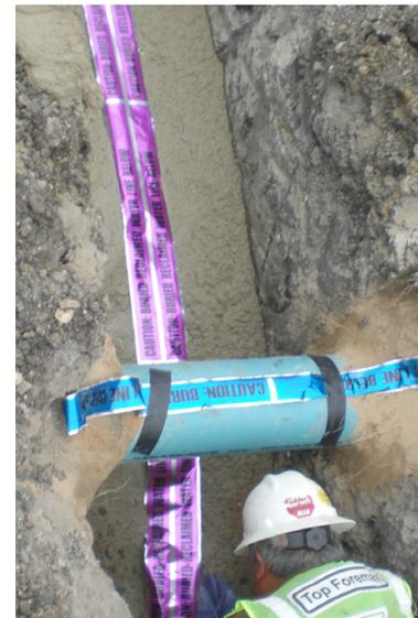
**Figure 10.5** Purple warning label indicating reclaimed water pipe buried below
