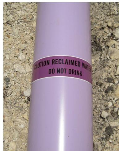
**Figure 10.1** Purple tape with integral label wrapped around pipe
