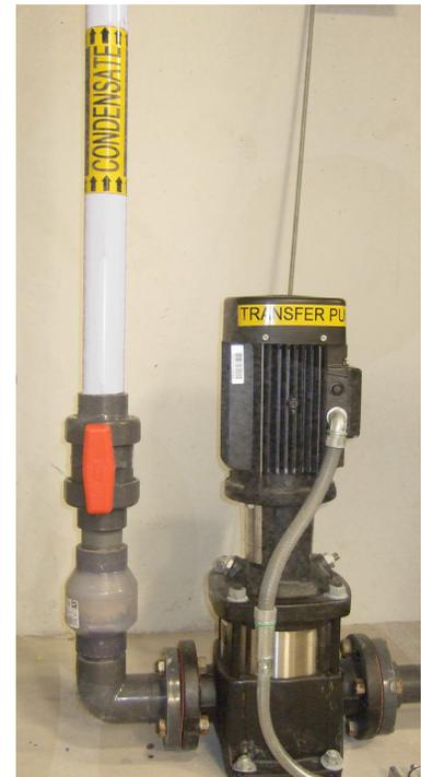
Figure 10.6 Condensate drainage pipe between AHU and storage tank
