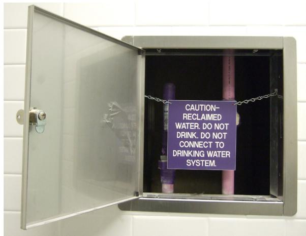
**Figure 9.16** Appurtenance access in building wall with door open and proper signage
