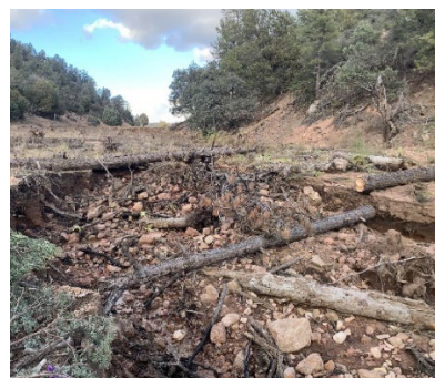
Figure 7: New headcut at bottom repaired in Phase 2
