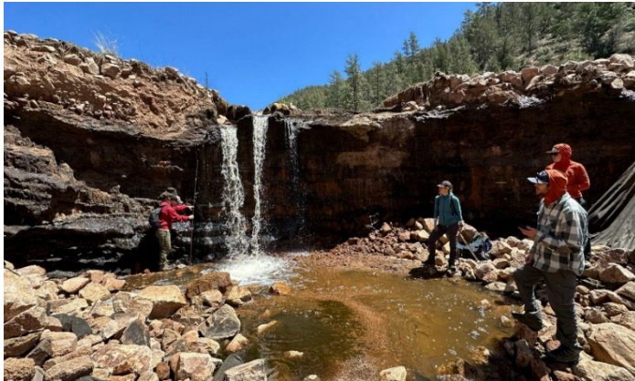
Figure 1: Most significant headcut in 2024 prior to restoration.
