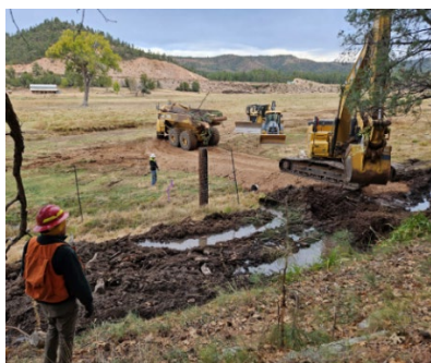
Figure 5: Building the access road
