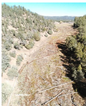
Figure 6: USFS drone footage of Phase 1 taken 12/2025 looking upstream
