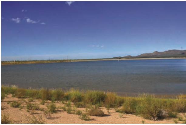
Figure 10.2 One of several groundwater recharge basins of the Southern Avra Valley Storage and Recovery Project (SAVSARP) used to recharge the aquifer with Colorado River water. Source: Artiola, Uhlman, Hix, 2017. Arizona Well Owner's Guide to Water Supply 2 nd Edition .
