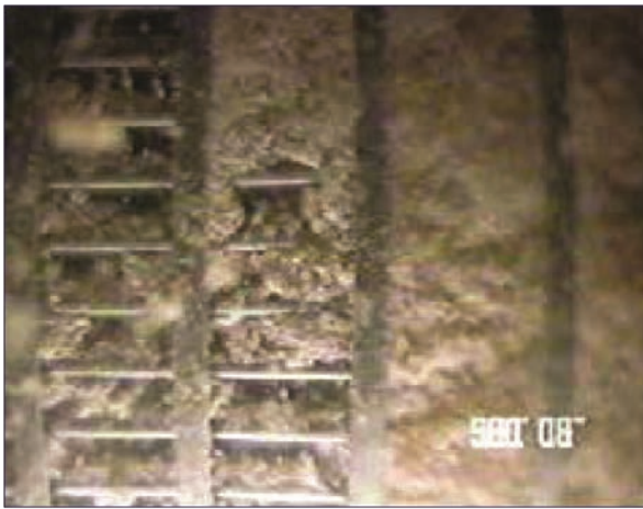
Figure 4.2 Scale formation on a well screen. Source: Artiola, Uhlman, Hix, 2017. Arizona Well Owner's Guide to Water Supply 2 nd Edition
