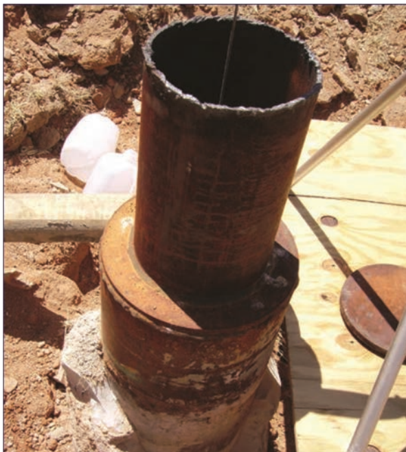
Figure 3.4 Photo of the sanitary seal grout around the surface casing of a well in construction. Source: Artiola, Uhlman, Hix, 2017. Arizona Well Owner's Guide to Water Supply 2 nd Edition
