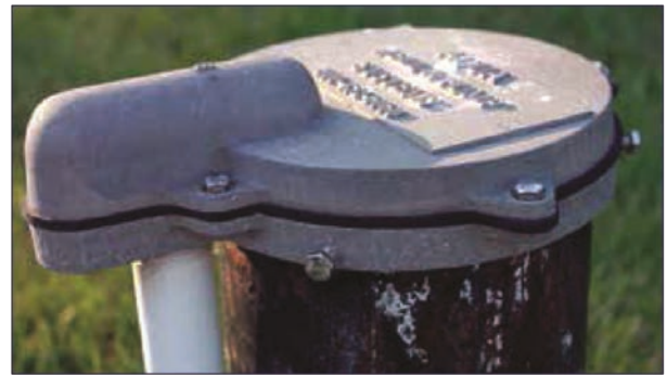
Figure 3.5 Example of a well cap made of aluminum. Source: Artiola, Uhlman, Hix, 2017. Arizona Well Owner's Guide to Water Supply 2 nd Edition
