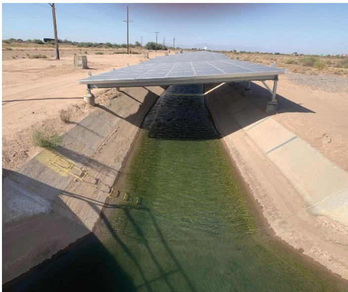
GRIC solar project—solar panels over canals. Source: Northeast Valley News
