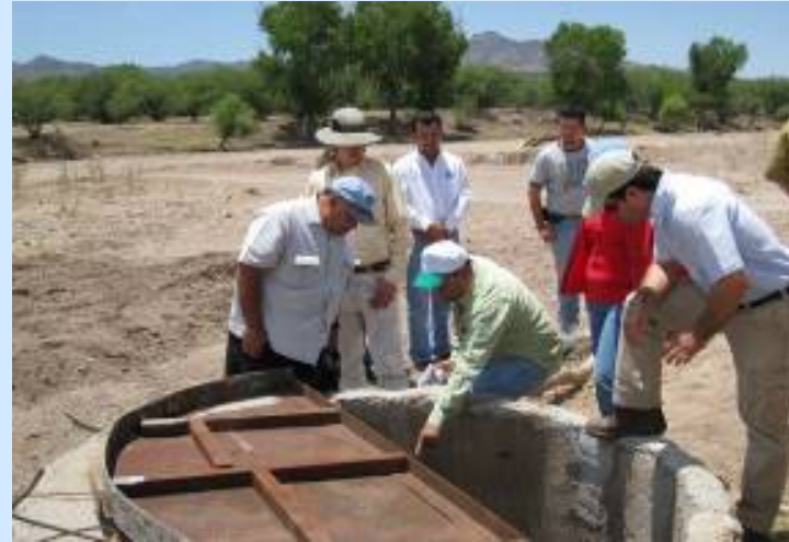
Paredes Infiltration Gallery, Mexico
