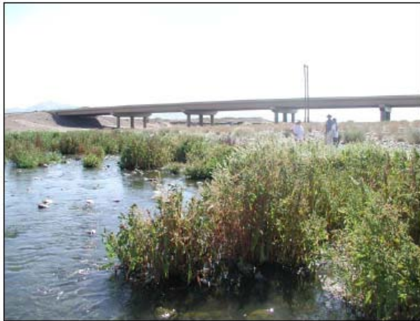
Low flow channel with wetland vegetation, immediately upstream of 51 st Avenue Bridge.
