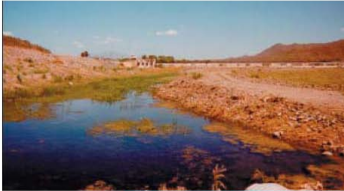
Water Seepage from Granite Reef Dam
