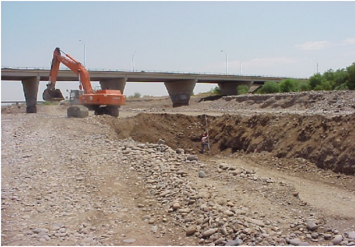
Construction of Low Flow Channel
