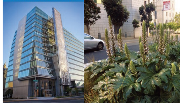
San Francisco Public Utilities Commission Headquarters – 525 Golden Gate Avenue
