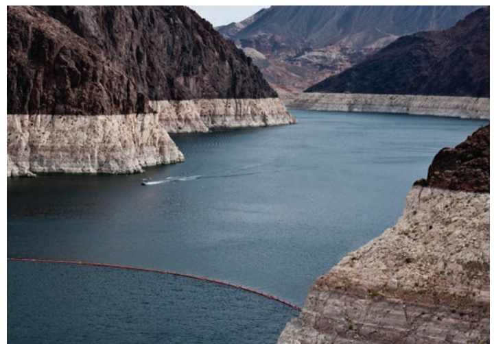
The "bathtub ring" showing decline in water elevations at Lake Mead. Source: National Aeronautics and Space Administration
